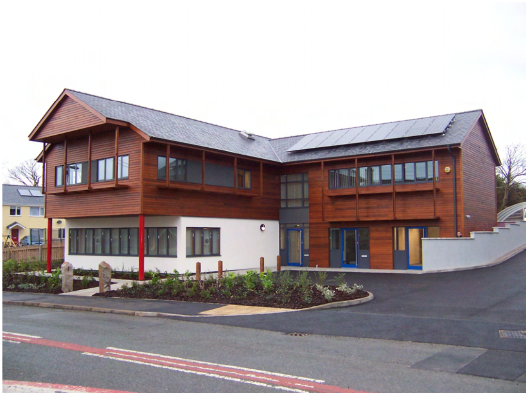
Figure 4.2: The new Enterprise Centre in Botwnnog
