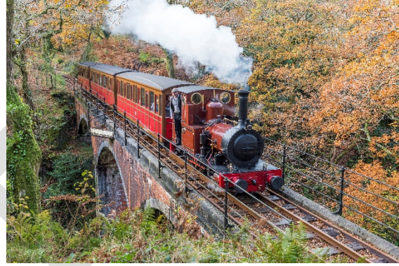
Talylyn Railway crossing Dolgoch viaduct (Component Part 6) © Rheilffordd Talylyn Railway
